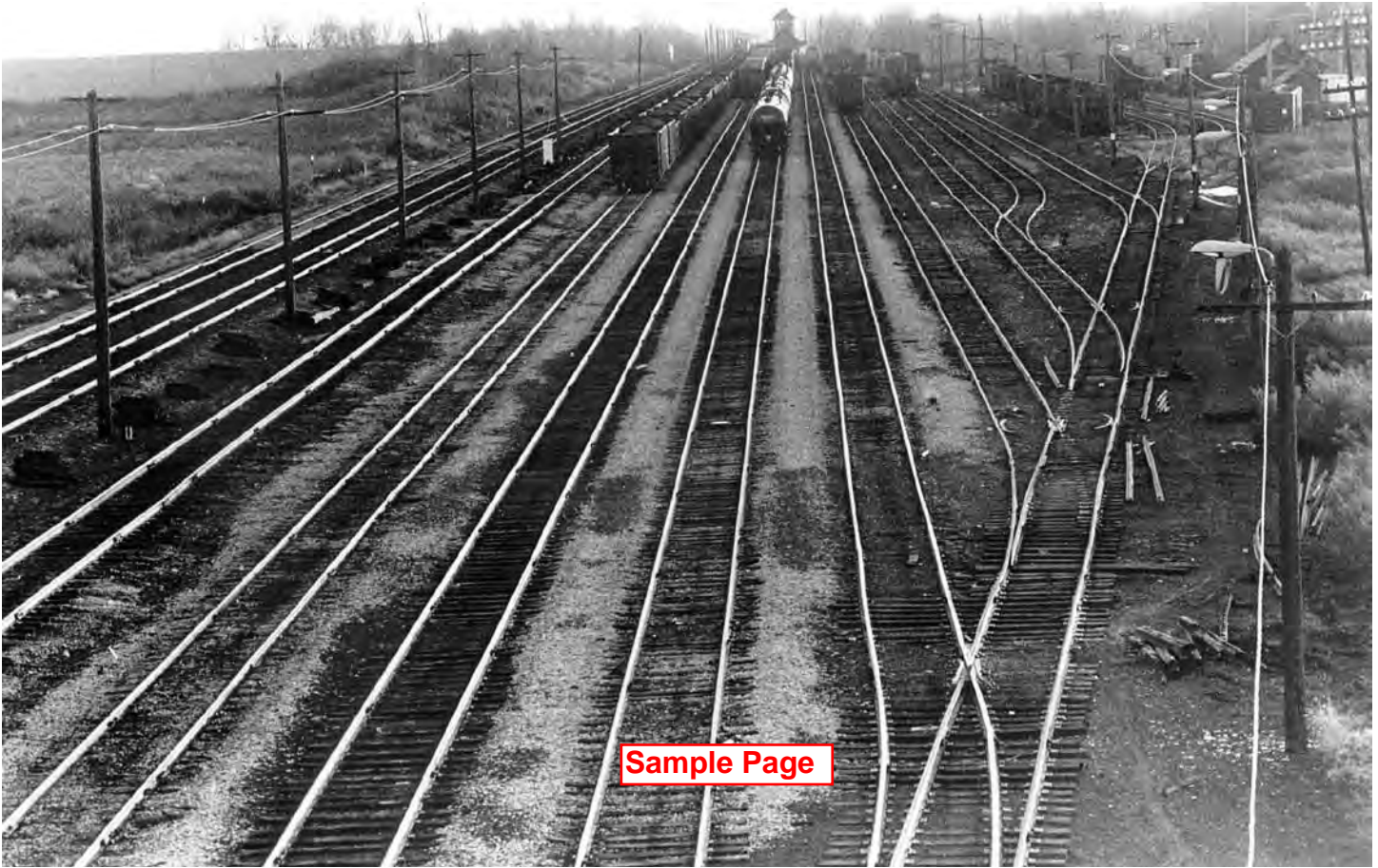
The yard at Brooks Avenue in Rochester, New York, was the BR&P/B&O's main sorting point for coal being shipped across Lake Ontario. The tall structure in the distance is the yard office. At one point the B&O could have as many as 700 loaded hoppers in the yard at Dock Junction or on the mainline past Rochester at Brooks Avenue. (Keith Pritchard collection)
