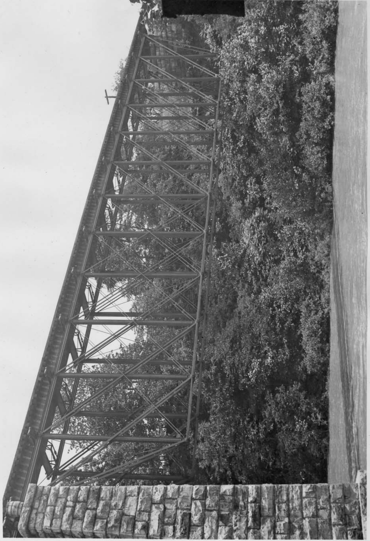
WHIPPLE TRUSS Br. No 120 Valley Railroad of Virginia Crossing North River of Cave Station, Va.
