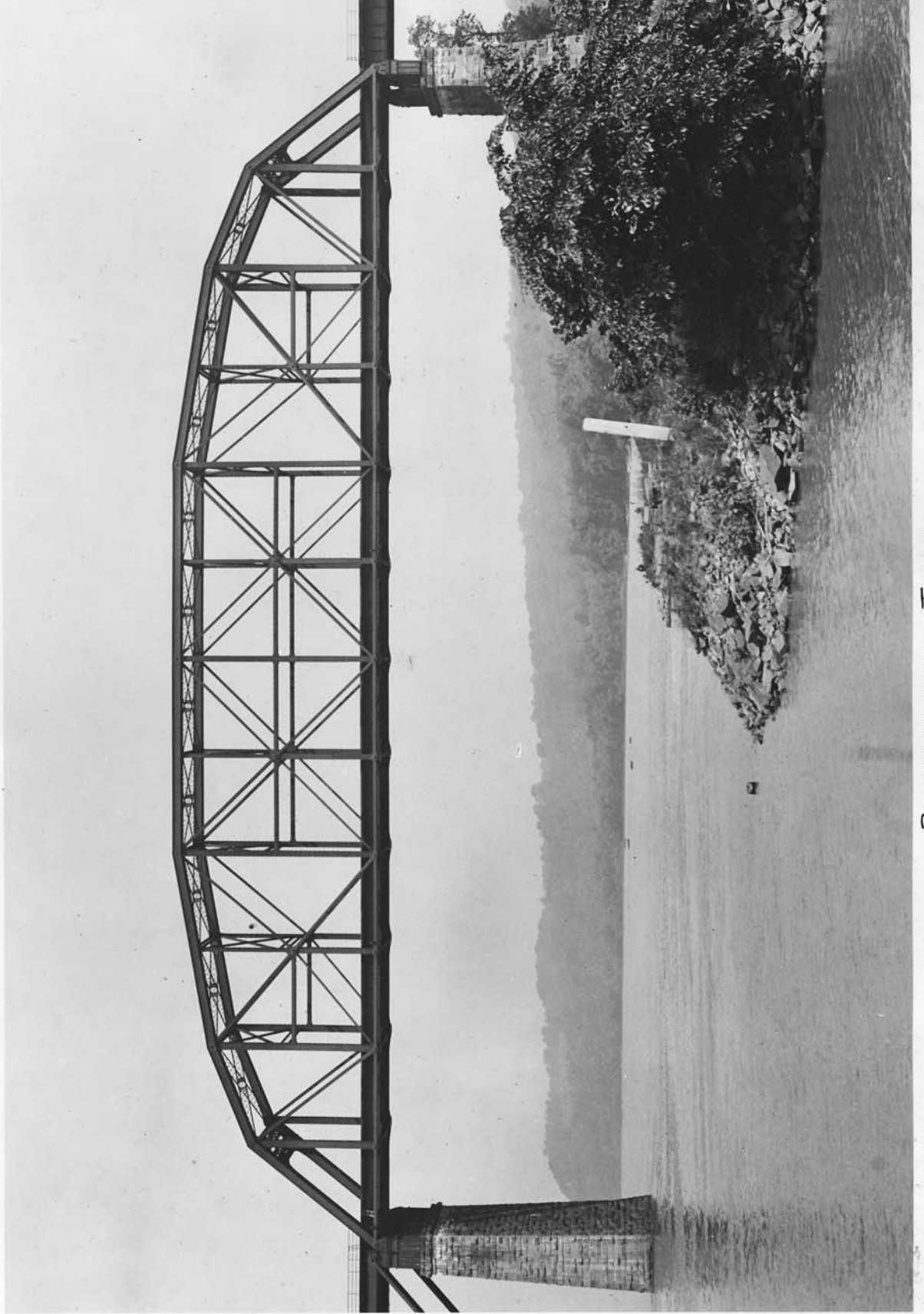
Br. No. 34A Philadelphia Div. - crossing East Channel of Susquehanna River at Havre de Grace, Md.
